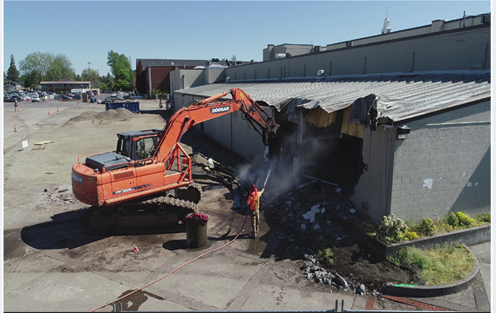
Demolition at North Salem High School in 2019
