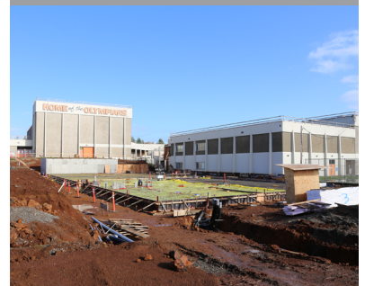
Southwest classroom addition
